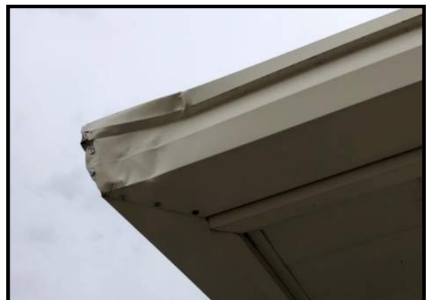
Image 18: Damage to gutter system at soffit
