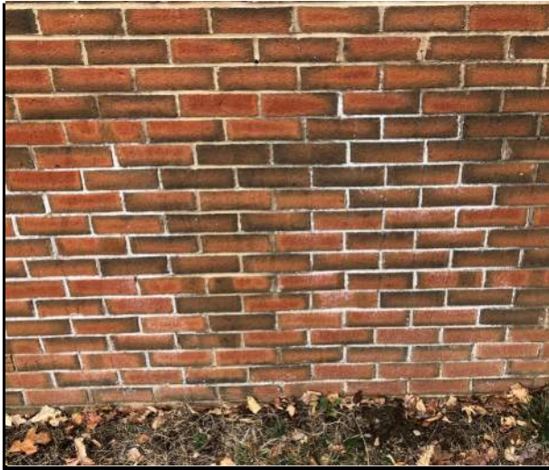
Image 7: Staining and mildew on brick
