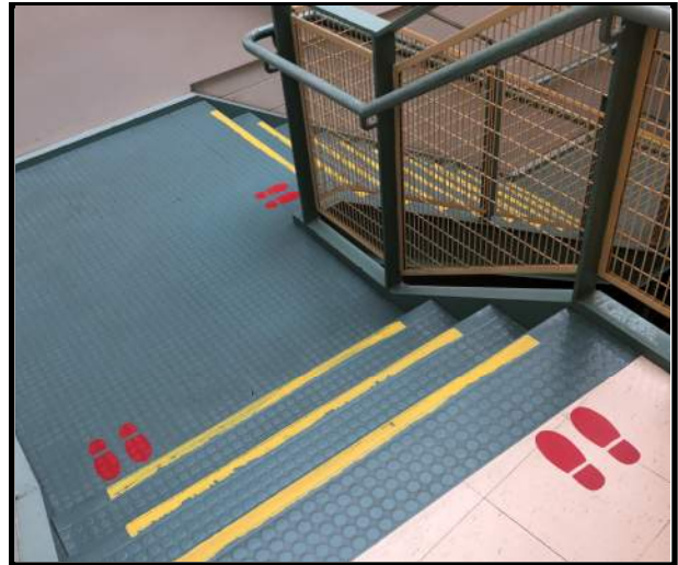
Image 10: Raised rubber flooring on stairway
