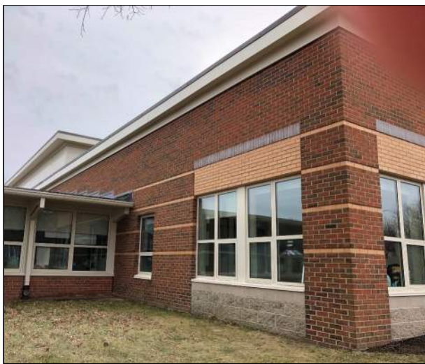
Image 5: 2003 addition brick and CMU pattern
