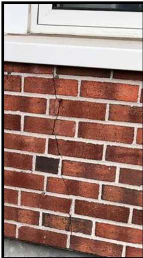
Image 9: Cracked Bricks
