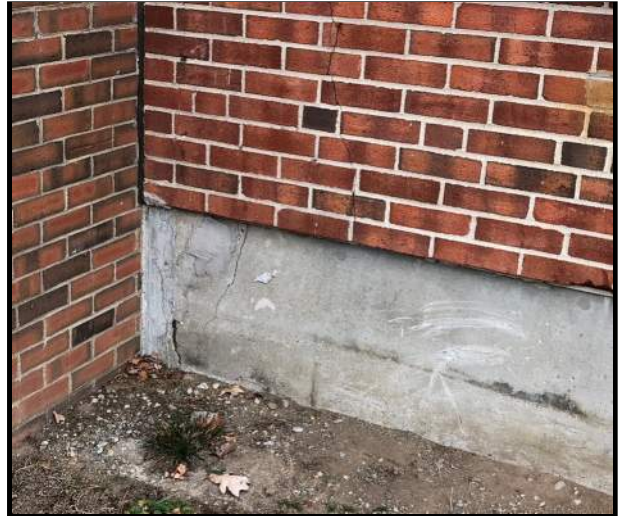
Image 2: Some foundation cracking in corner
