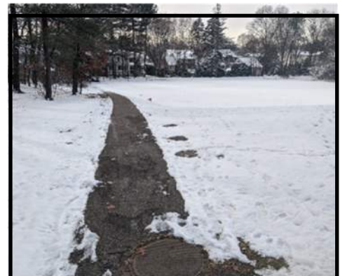
Image 15: Tear parking lot sheet flow to field
