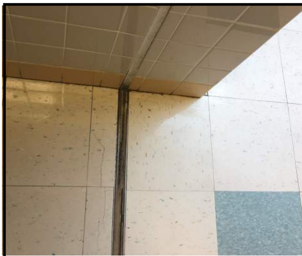
Image 5: Damaged flooring at transition
