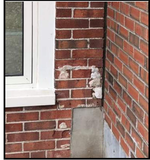
Image 10b: Excess grout on walls
