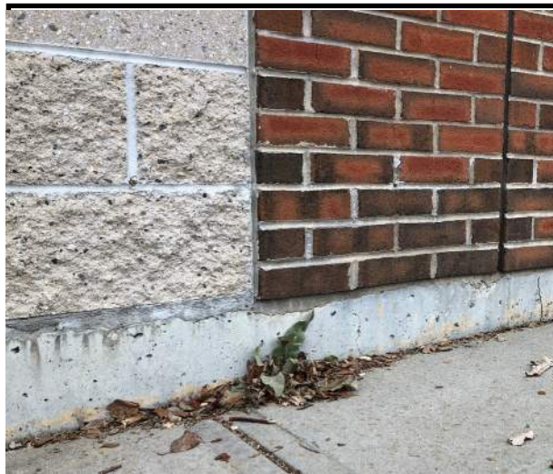
Image 3: Spalling concrete at joint
