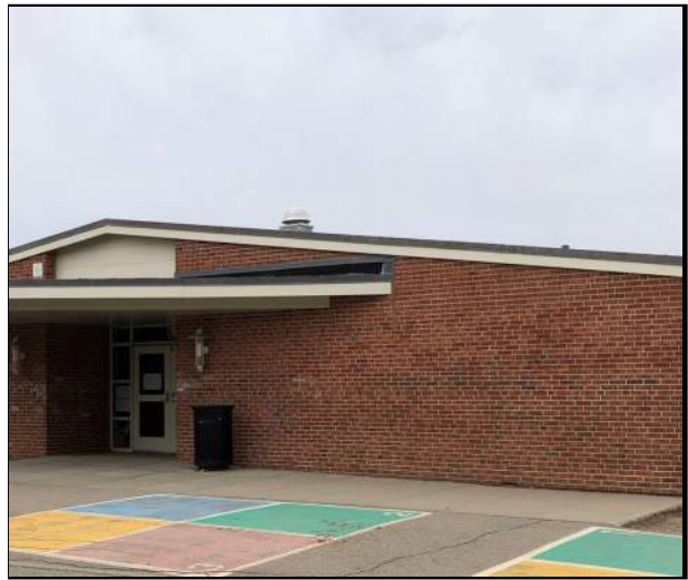
Image 4: Original brick with Flemish bond course
