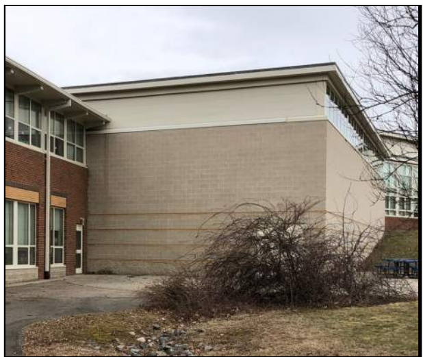
Image 6: 2003 addition with CMU and glazed brick
