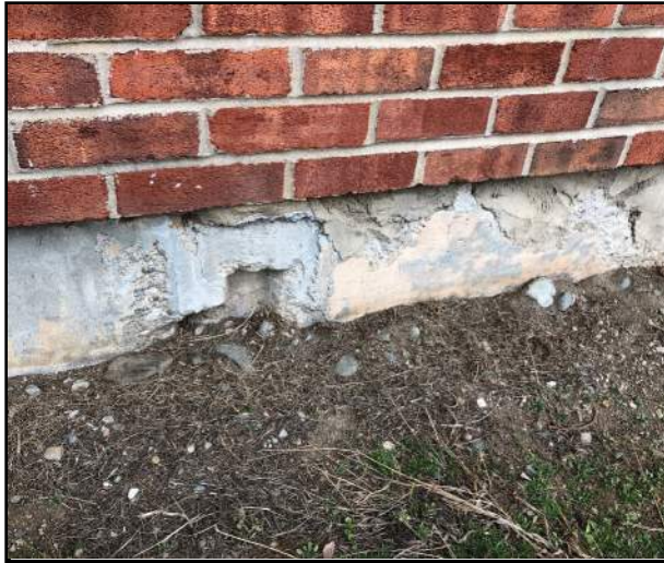
Image 1: Previously patched foundation area
