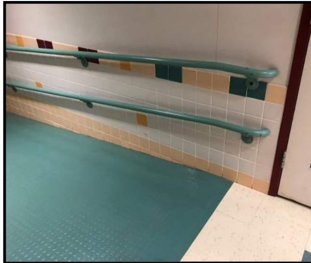
Image 9: Raised rubber flooring at ramp
