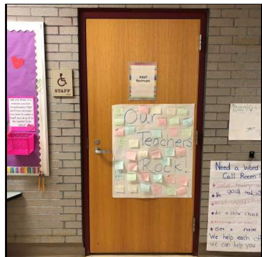
Image 22: Typical solid WD door and HM frame
