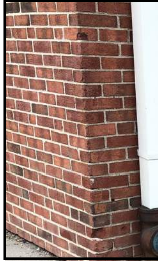
Image 10a: Damaged Bricks
