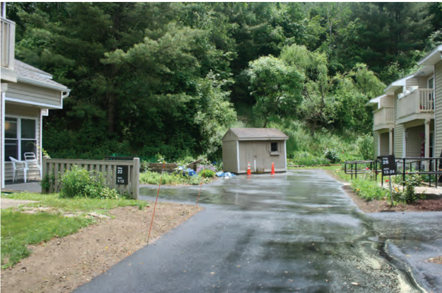
5. Apartments between buildings have asphalt drives that dead end into hillsides. They facilitate emergency vehicle access and accessibility, but add to the amount of paving on the site.
