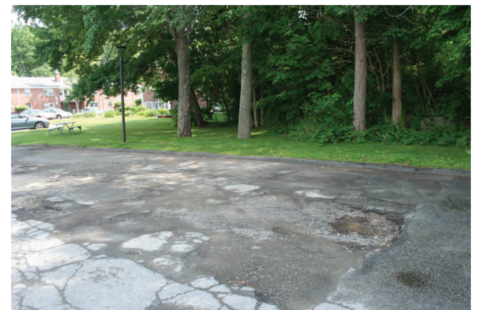
12. Paving is in poor condition, and the site is undeveloped in terms of offering resident amenities. The surrounding trees and topography shelter the Chambers Street buildings from the surrounding neighborhood. Recent paving has improved some areas.
