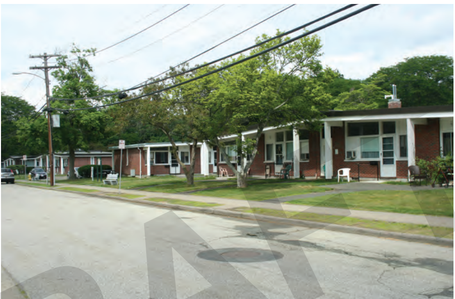
2. Half the buildings are oriented parallel to the street and half are oriented at 90 degrees, forming a kind of basket weave pattern in the overall layout. The brick buildings have overhanging roofs on both sides supported by steel columns clad in white painted wood.
