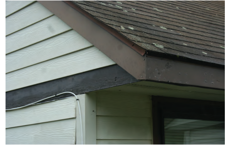
12. Roofs, eaves, soffits and trim are all in relatively poor condition. Their construction is similar to Seabeds, which suffered damage from ice dams in 2015 requiring $1.6 million dollars in emergency repair funding.
