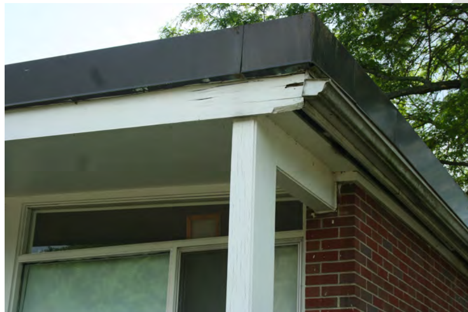
10. Buildings are in relatively good condition. Roofs were replaced in 2018. Masonry is in good shape. Some of the wood trim and windows need to be replaced.
