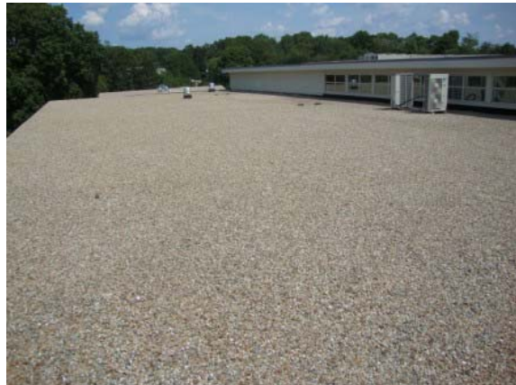
Photo #22: Four ply built up roof system with flood coat and Aggregate Surfacing
