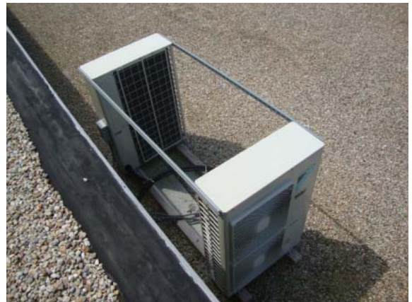
Photo #12: Split system air conditioning units for cooling data centers
