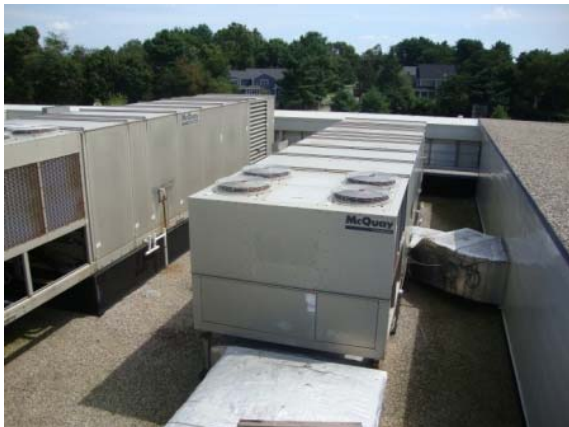
Photo #11: Five McQuay rooftop cooling units (RTU) with natural gas furnace
