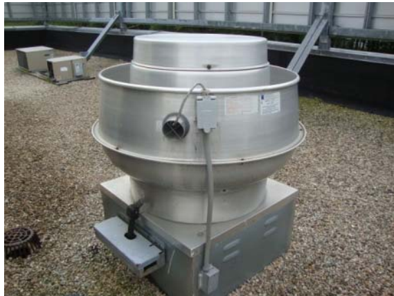
Photo #39: Kitchen vent discharge
