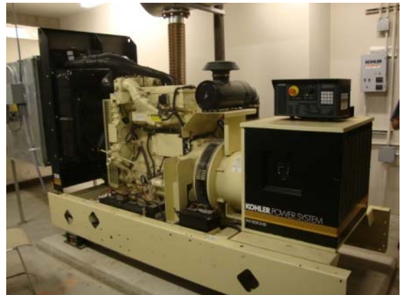
Photo #18: Kohler diesel generator
