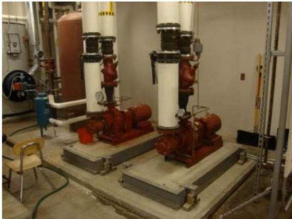
Photo #9: Hot water recirculation pumps
