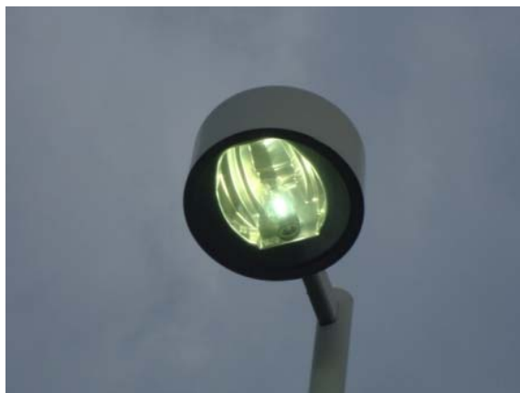
Photo #41: Exterior metal Halide pole lights
