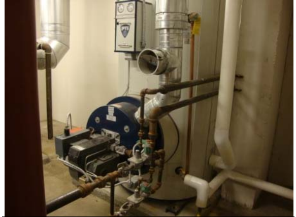
Photo #8: Buildings hot water heaters
