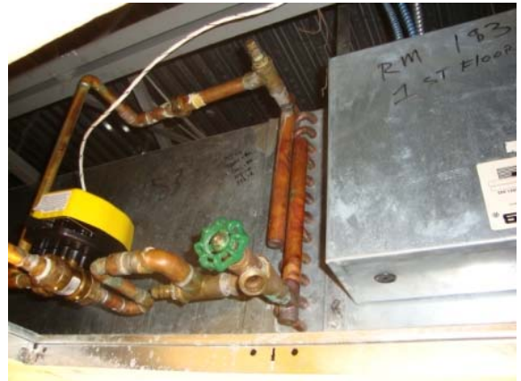
Photo #10: VAV boxes in the ceiling of rooms
