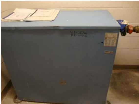
Photo #21: Elevator oil reservoir with submersible sump pump
