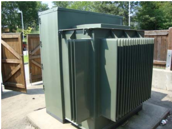
Photo #17: Pad-mounted transformer
