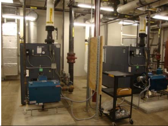
Photo #7: Two Weil McLain Boilers - providing heat to building
