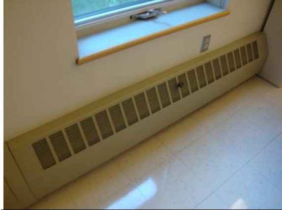
Photo #20: Baseboard hydronic heating unit on exterior walls of rooms
