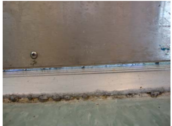
Photo #40: Space under door at north end emergency exits - 2 doors (needs door sweeps)
