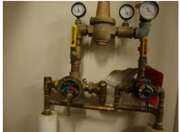
Photo #16: Mixing valve for buildings hot water
