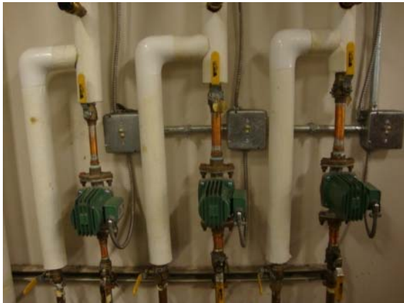
Photo #15: Domestic hot water recirculation pumps
