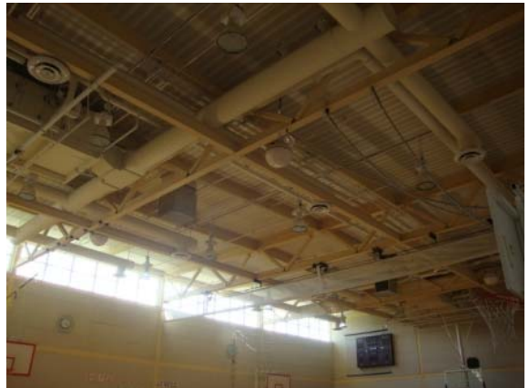
Photo #34: Gym has sufficient day lighting to avoid using 400W metal Halide lights
