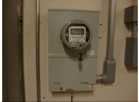
Photo #14: Main electric meter for building
