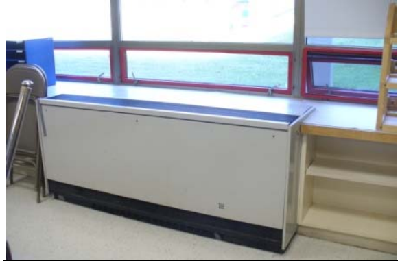
Photo #26: Typical unit ventilators
