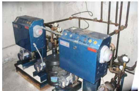
Photo #18: No.2 oil pumps for the boiler
