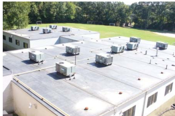
Photo #22: Packages RTU's serving the portables
