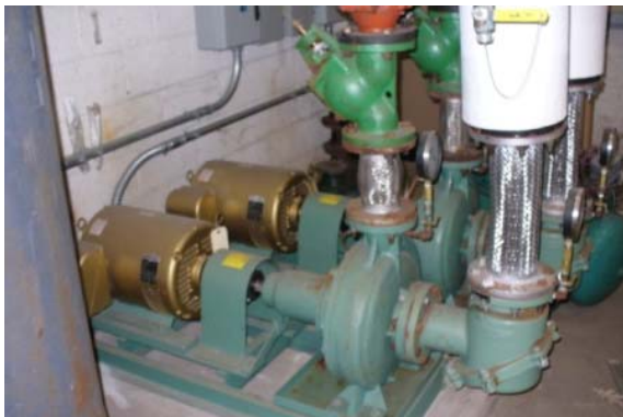
Photo #21: Hot water circulation pumps in Boiler Room 2
