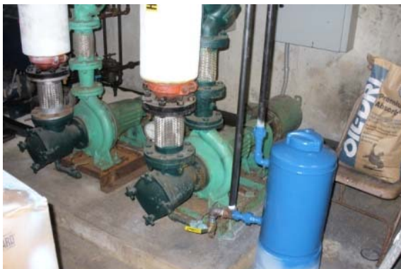
Photo #17: Main hot water circulation pumps
