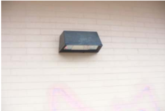
Photo #37: External wall pack with 40W CFL
