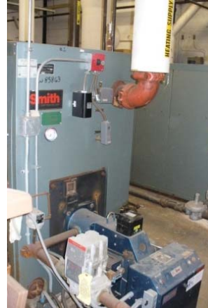
Photo #20: Hot water boilers in Boiler Room 2
