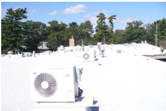
Photo #23: Roof top split systems serving individual spaces
