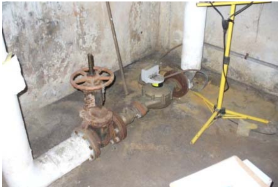
Photo #15: Main domestic water meter
