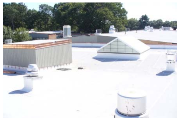
Photo #24: New flat roof and skylights
