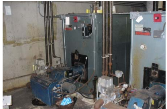
Photo #16: Natural gas-fired hot water boilers in the front boiler room
